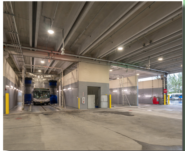
Ravenswood Bus Maintenance Facility Dania Beach, Florida
