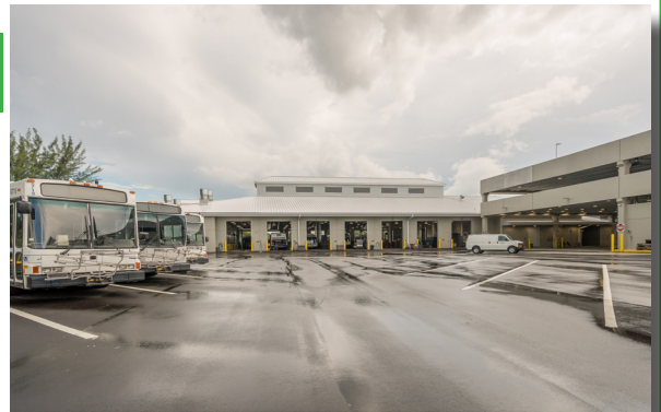
Ravenswood Bus Maintenance Facility Dania Beach, Florida
