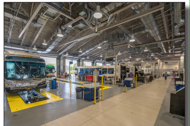
Ravenswood Bus Maintenance Facility Dania Beach, Florida
