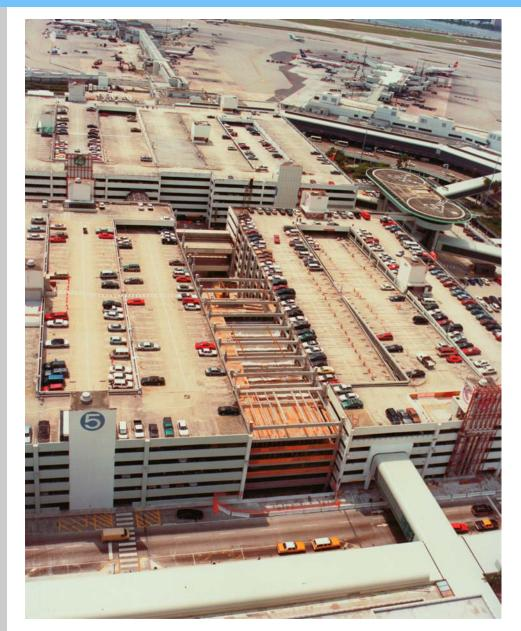
A seven story' vehicular parking structure infill between two active public parking garages at Miami International Airport. The 65' x 400' concrete structure introduces 400 additional parking spaces to the MIA revenue parking environment.
