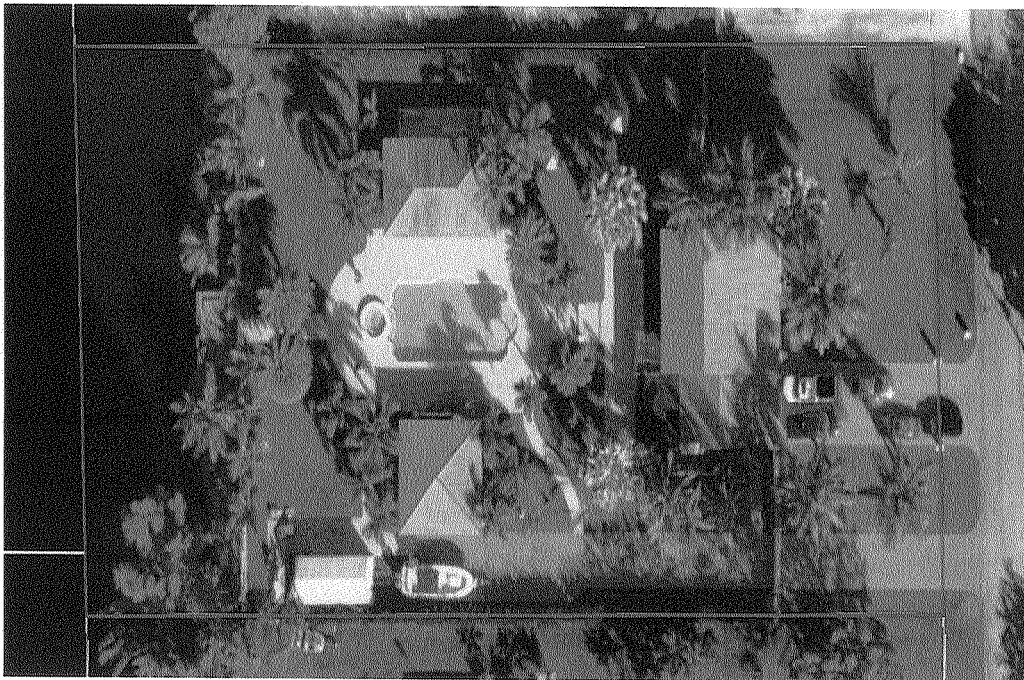
Location #8: 3850 S.W. 137 th Avenue, Miramar
